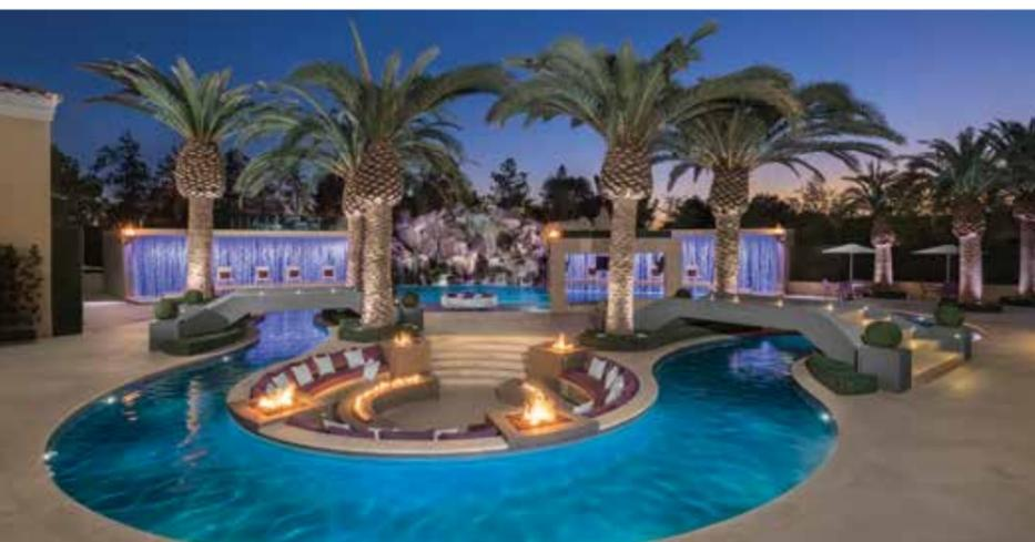
Above: This dramatic water wall stands 10 feet high and spans 40 feet in length. Basalt stone lies behind the curtain of water while large slabs of limestone provide surface area for seating. The interior of pool itself is built of beadcrete, and features a swim-up bar on the far right. Designed and built by Red Rock Pools and Spas.
